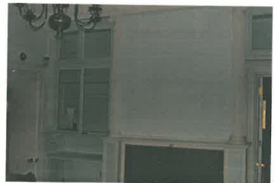
Wood trim that was covered by coats of old lead paint, right , was stripped bare, revealing the original wood detail, above . Dental picks were used to remove every trace of the paint.
