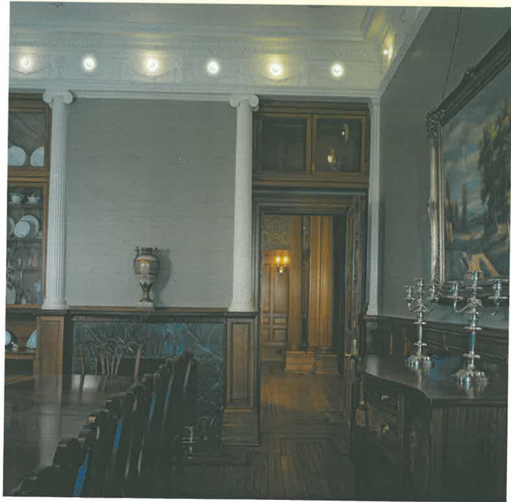
Wood trim that was covered by coats of old lead paint, right , was stripped bare, revealing the original wood detail, above . Dental picks were used to remove every trace of the paint.
